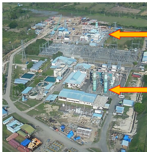
Aerial view of Sengkang Power Plant
